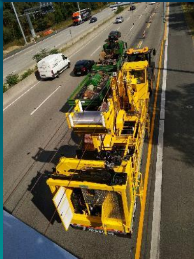
Pulling the contact wire
