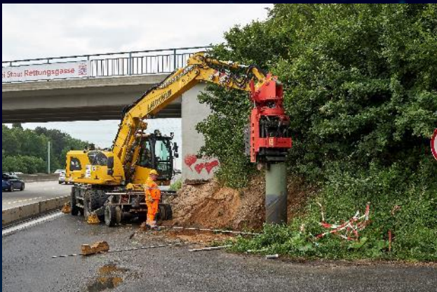
Rammed the steel pipes
