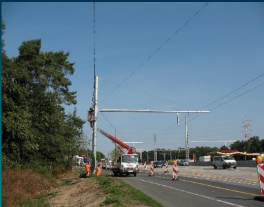
Attachment of the cantilevers
